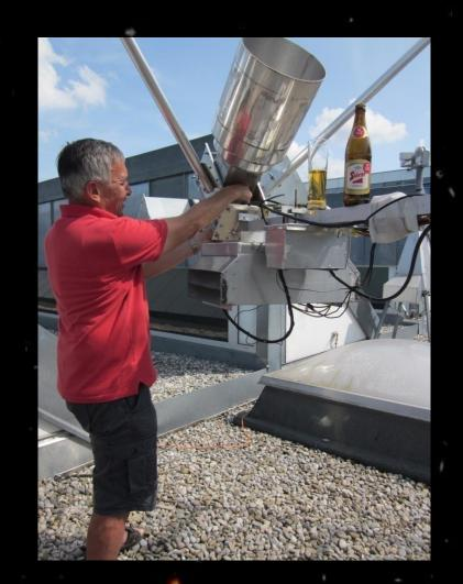
....adding/removing feed is easily done within 10 minutes 70 cm dual dipole feed...and with weather protection
